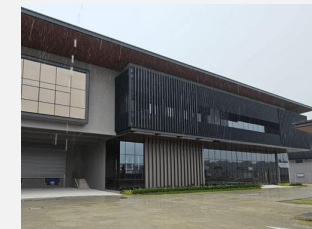
Malaysia Operations Center (being constructed)
