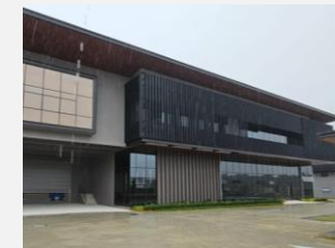
Iskandar Puteri, Malaysia Operations Center (being constructed)
